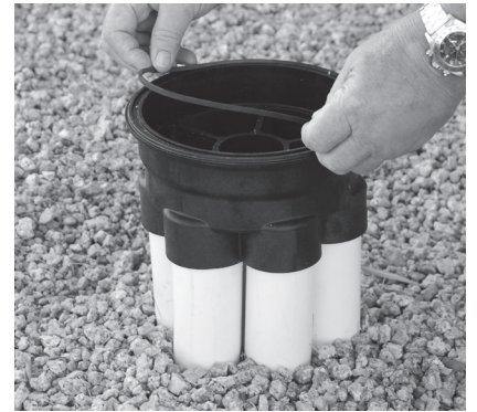
3. Clean and install base o-ring
