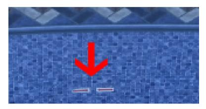
We do not faceplate until there is proper water pressure on the fittings to ensure our gaskets are properly sealed. It is not unusual for water to be over the lights, returns, skimmers, etc. before we faceplate. These arrows show our face plating process. Expect the liner to be covering these areas until we install their faceplates.
