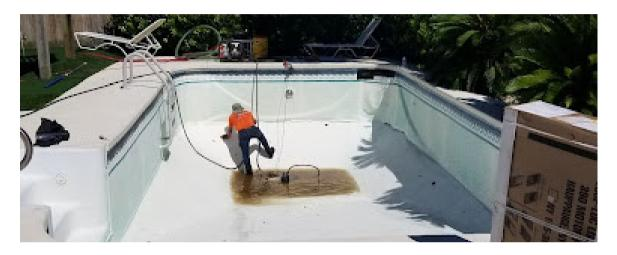
Our liner replacement team will come out before the liner is installed to properly drain the pool. They will use the wellpoint, if there is one, to alleviate the groundwater. Once the pool is fully drained and dewatered, we will remove the liner and start the prep work.
