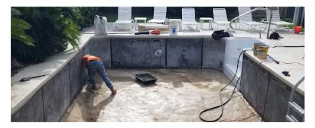
Once the pool is empty, the old liner and debris can be removed. We will asses for rust on steel walls, algae growth on the pool floor and damage to the pool floor that was not visible when liner was in place.
