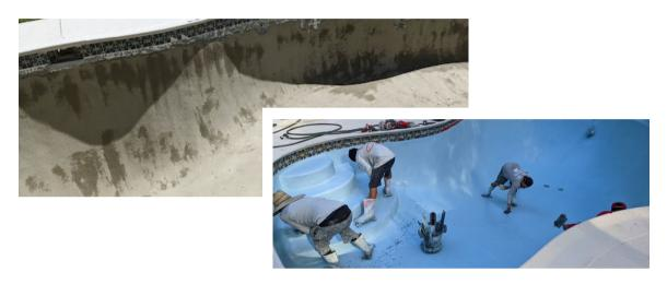
Our plaster crew will come out to prepare your pool for plaster once the tile is completed. During this process, all fittings are waterproofed around the penetrations, and new fittings will be installed where necessary. The plaster process typically takes up to 48 hours to complete based on size and select finishes. Once the plaster has been installed, our team will start filling the pool while using a sequestriant to help with the curing process.
