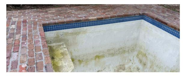
The size of the tile used in the pool renovation is determined during the material selection process. Most of our clients prefer a 6"x6" or 6"x12" tile. The removal and installation of the tile usually takes 2-4 days, depending on the amount of tile that needs to be installed.
