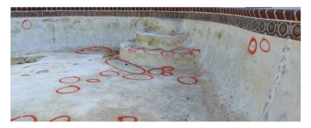
After our team has fully drained your pool, one of our service technicians will sound the pool for hollows. This process involves using a hammer to listen for hollow areas in the plaster. By doing so, we can determine if the pool needs to be fully chipped to remove the surface, ensuring that the new plaster will properly cure and bond.
