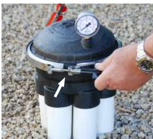
8. While tightening band clamp, lightly tap clamp with a screwdriver or wrench. 1/2" gap once tightened.
