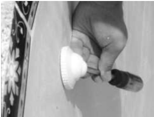
Proper Positioning Of Down Jet Eyeball
