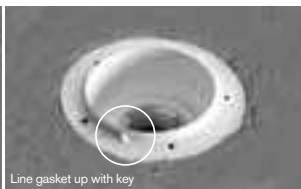
Line gasket up with key
